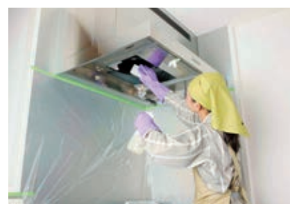
Cleaning of extractor fans
