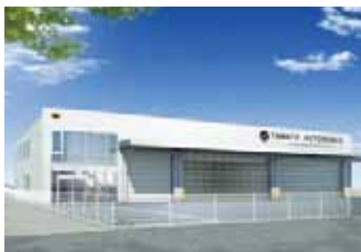
Superworks Gunma vehicle maintenance plant: completed in October 2011
