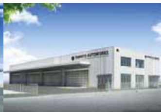
Superworks Saitama vehicle maintenance plant: to be completed in January 2012
